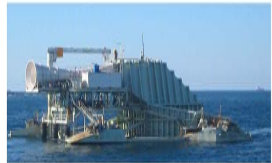
Oscillating Water Column Oceanlinx
