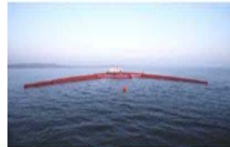
Overtopping Wave Dragon
