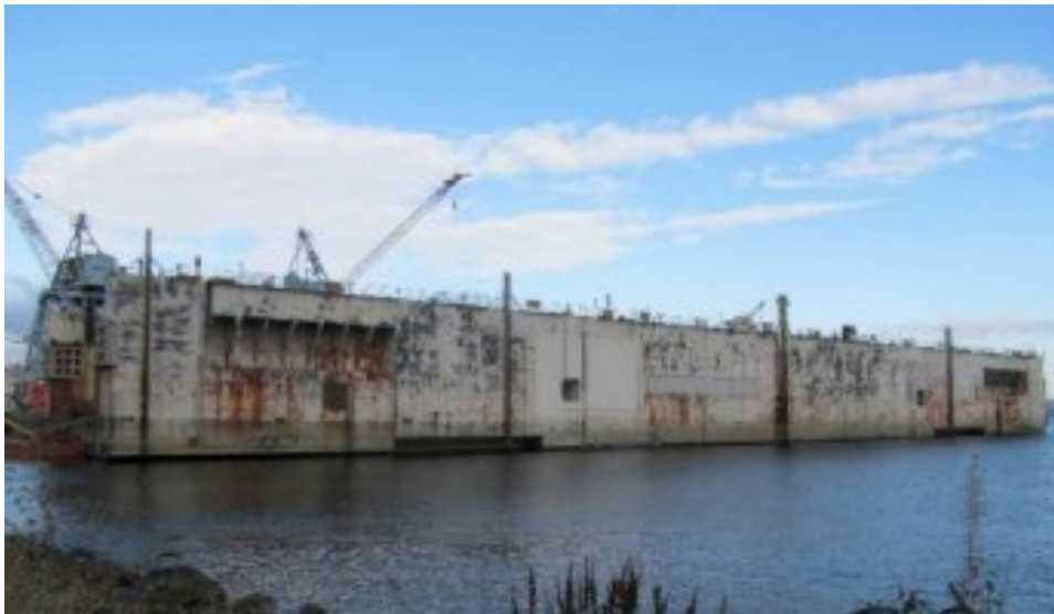
Figure 1. Starboard side of the YFD-70. Photo: Marine Surveyors & Safety Consultants, Trip in Tow Suitability Survey, Seattle WA. Dated August 2, 2016.
